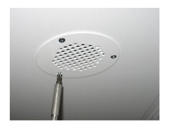
During Kwik-Kit installation you will be prompted to return to the KK-C-VAK instruction to attach the hose to the vent adapter brackets. Route hose into ceiling holes and <u>cut off any extra slack</u>. Attach the hose to the vent bracket using a 3" hose clamp
